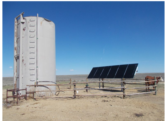
A new installed solar system on an existing livestock well.
