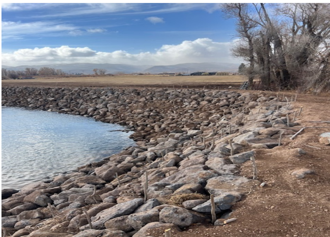
A portion of the Smiths Fork River eroding riverbank was shaped and rock-riprapped to curtail severe bank erosion
