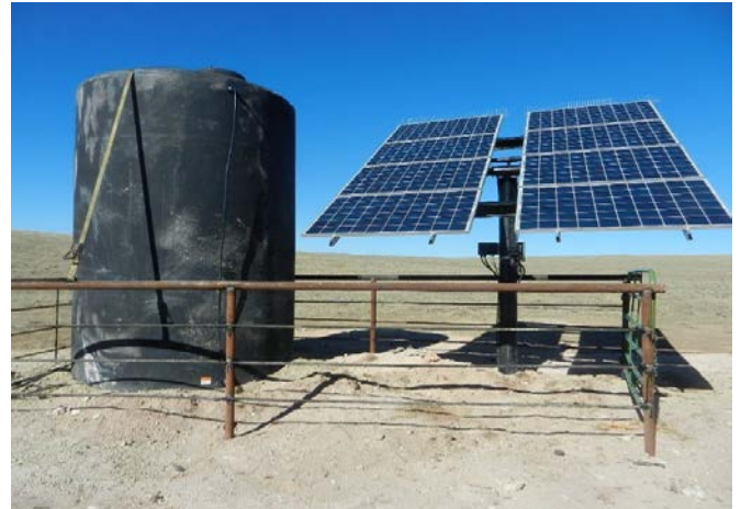
Storage tank and solar panels that were installed in south Lincoln County to help provide reliable water for livestock.
